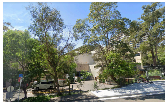
Image 1.5 Edgecliff Centre Loading Dock and right of way access to Eastpoint
