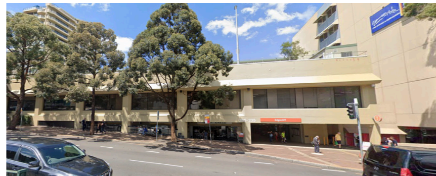
Image 1.3 Eastpoint and entrance to Edgecliff Railway Station
